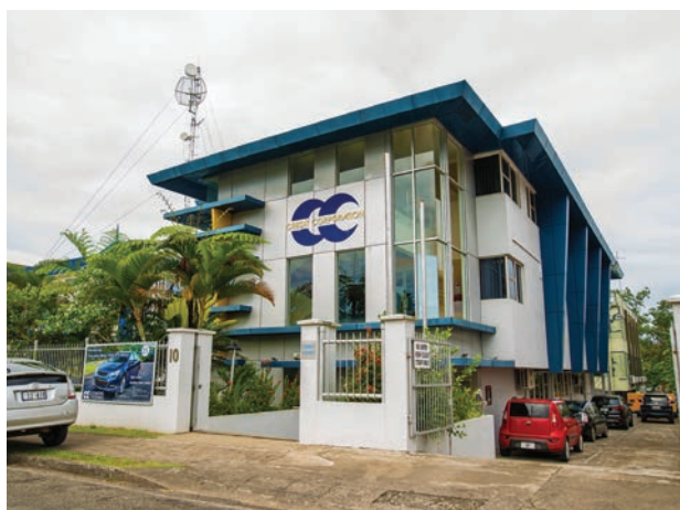
Suva Office, Fiji.
