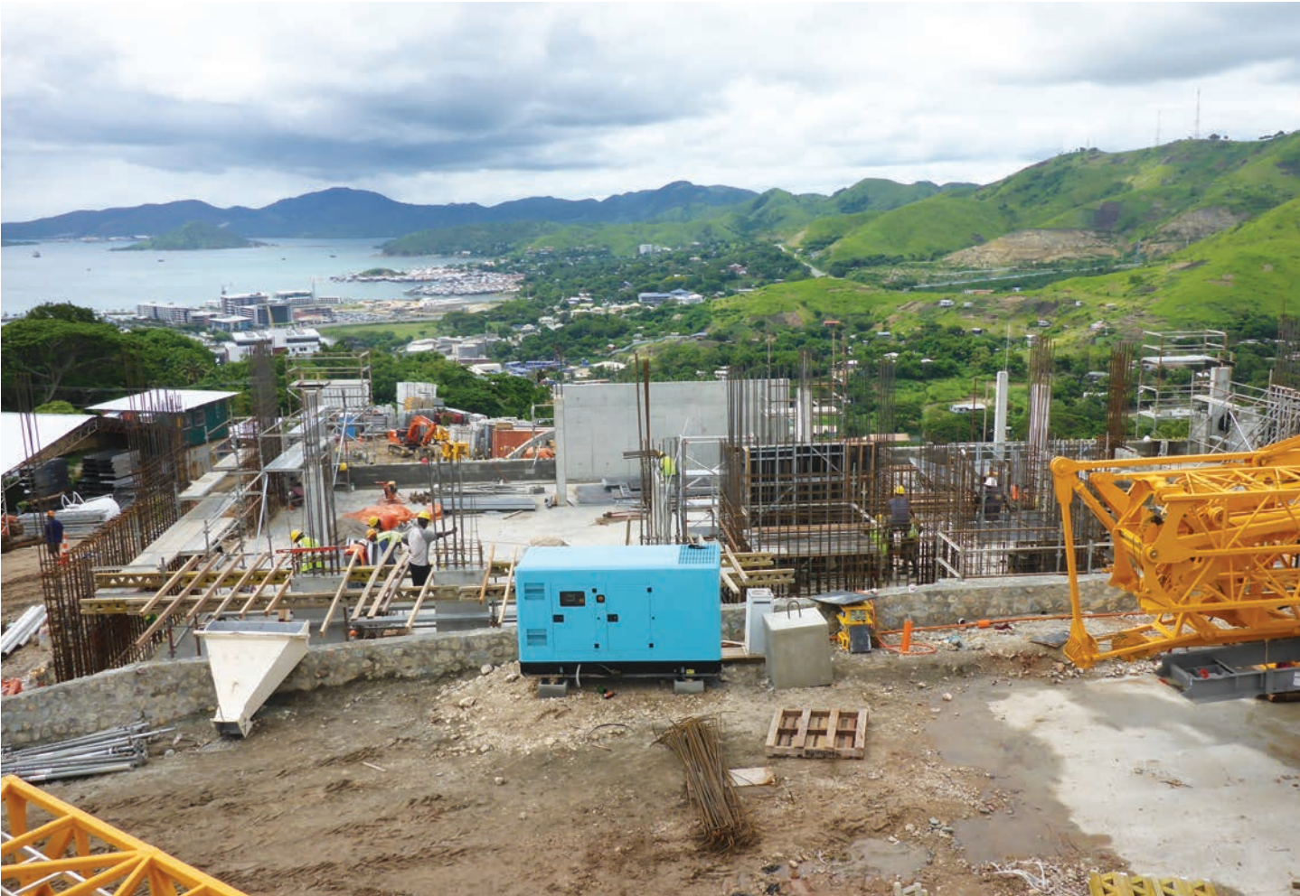
Ela Makana Project construction commenced.
